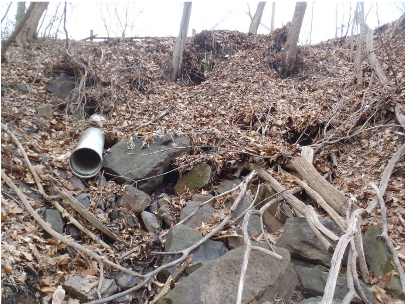
Photo 5: Large Stone Rip-Rap at Outfall
