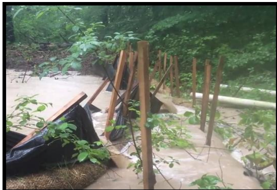
This silt fencing was not properly maintained, resulting in failure and discharge of polluted stormwater to the City's waterways.
